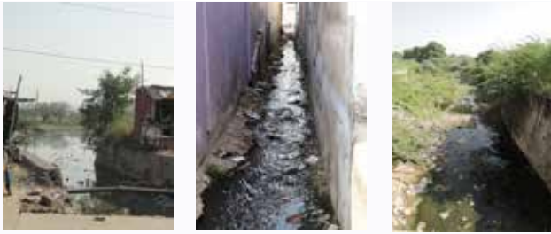
Condition of Drains in the city
