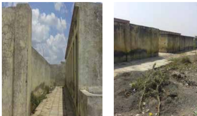
Old toilet blocks
